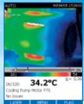
Cooling pump running at operating temperature.
